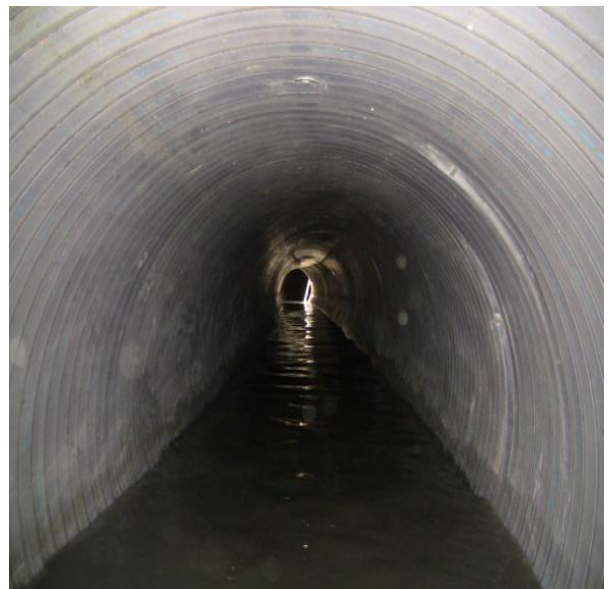
Rehabilitated pipe in HCMC
